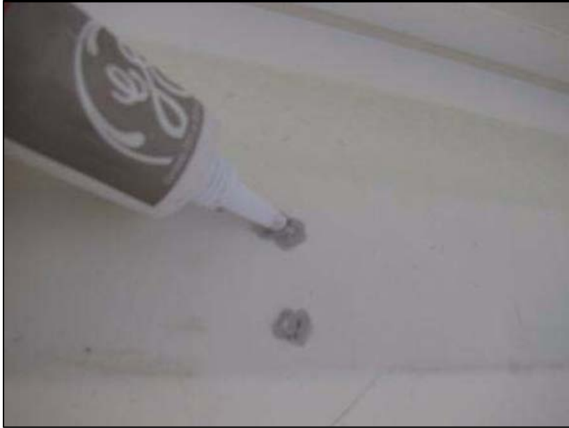
Figure 16: Sealant Applied to Backside
