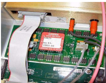
Figure 6 Connecting the Vcap and Vchamber cables to the power supply.
