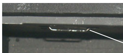
Bracket inside top of firebox.
