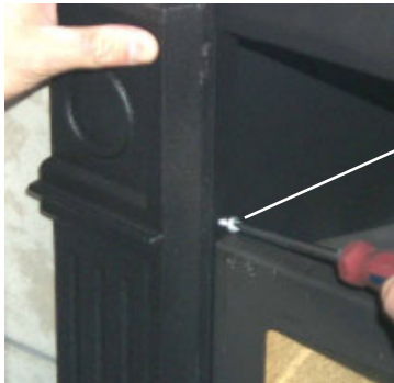
Secure top of faceplate with screw.
