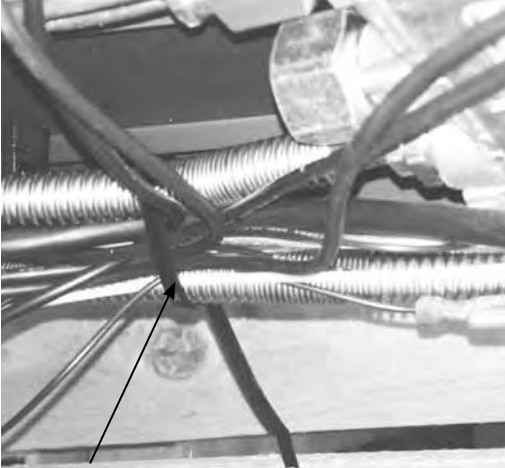
One of the tie wraps which secure the line set. Figure 14.
