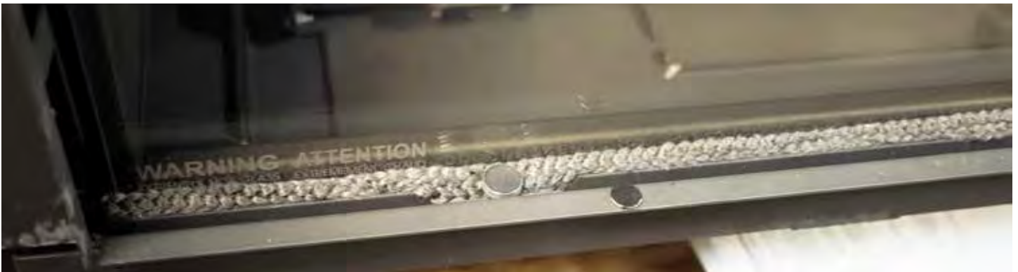
Figure 53 Place a single magnet on the bottom return flange 12" from the lower left corner, lower right corner, and the center.
