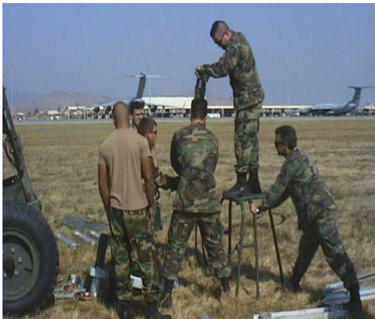
Figure A1. Driving Stakes from the MAAS Work Stand
