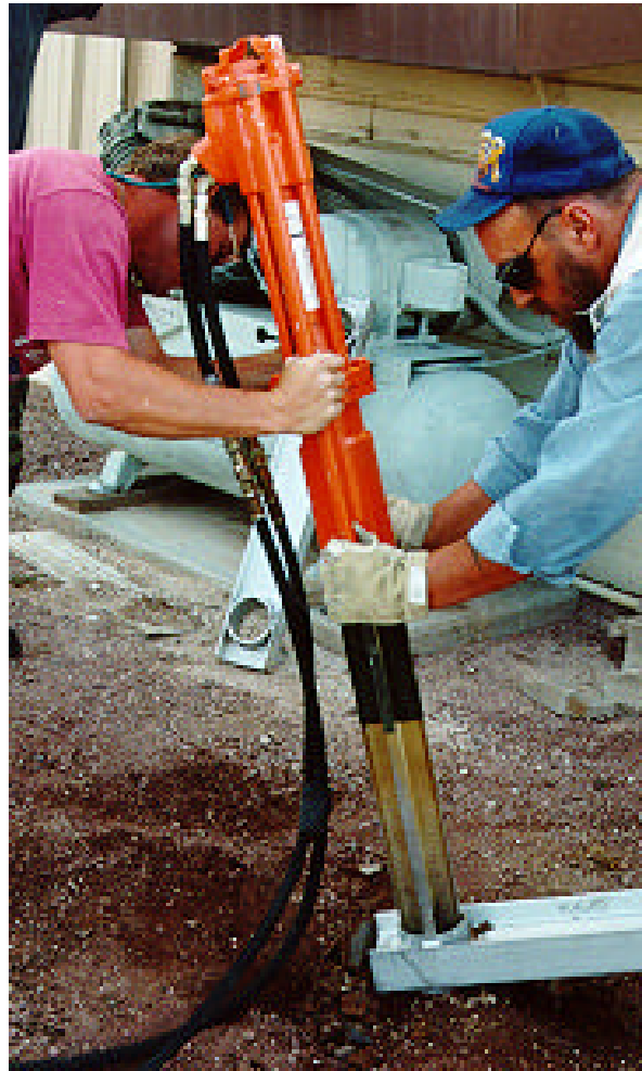
Figure A2. Driving Stakes Using the PD48142
