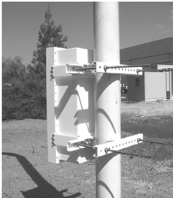
**Figure C-4. Rear View of Converter Installed on Round Pole**
