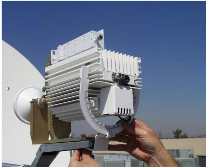
**Figure C-6. Installing the SSPA**
