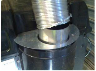
3/ Form extra bends where required. Care should be taken when forming bends to not create a low point where condensation may collect. Condensation should be able to drain to the heater or out the flue outlet. The flue should be bracketed at intervals of 1 M using standard 125 mm standoff brackets available at most plumbing suppliers.
