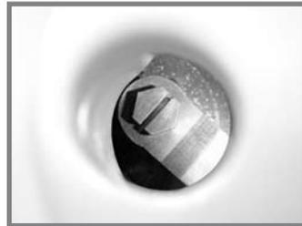
3. Insert screwdriver or 7/16-in. socket through access hole and onto hex head.
