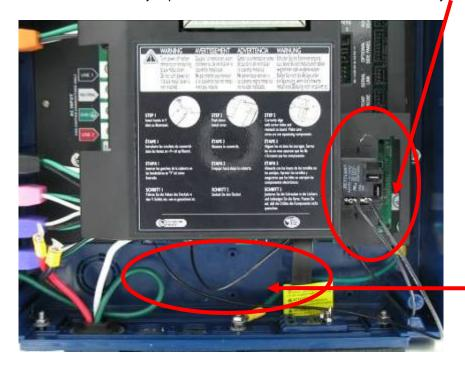
7) Connect the wires from the gas heater safety circuit to the relay terminals marked NO and COM
