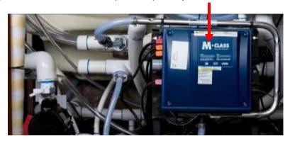
3) Attach the relay to the black shield in the Lower Control with two dots of silicone: one on the bottom and one on the side.
