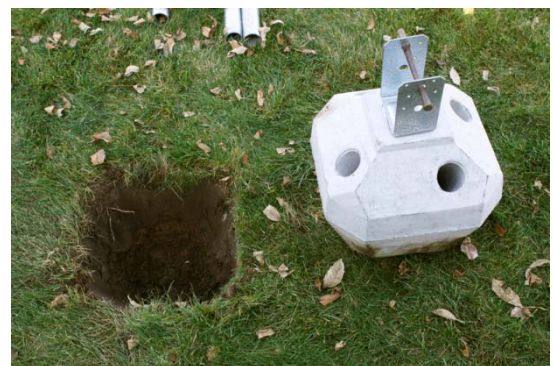
Figure 3. Tapered Hole for Concrete Head
