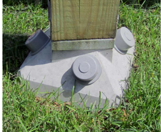
Figure 7. Completed Installation with Inspection Caps
