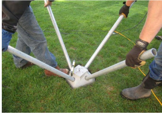
Figure 4. Setting Pins and Leveling Pier
