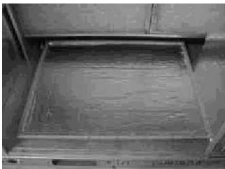
Figure 18: Return Downflow Plenum With Panel
