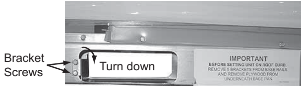
Figure 1: Unit Shipping Bracket
