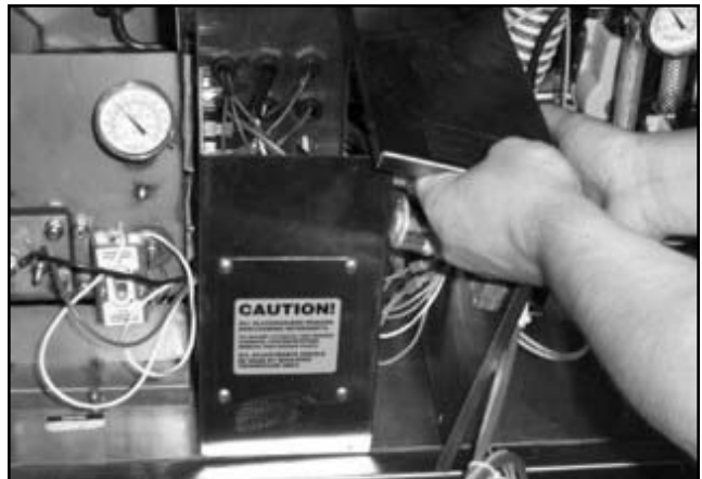
Removing the electrical box cover.
