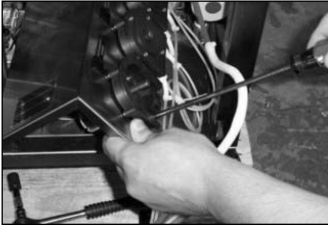
Removing the motor mounting screws.
