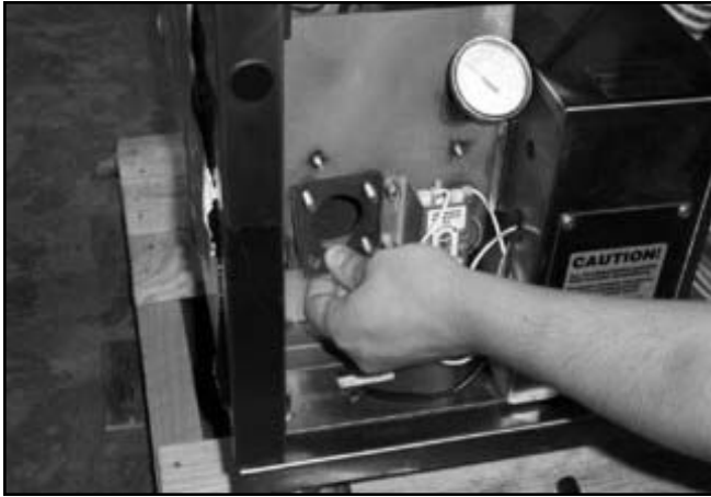
Removing the heater gasket
