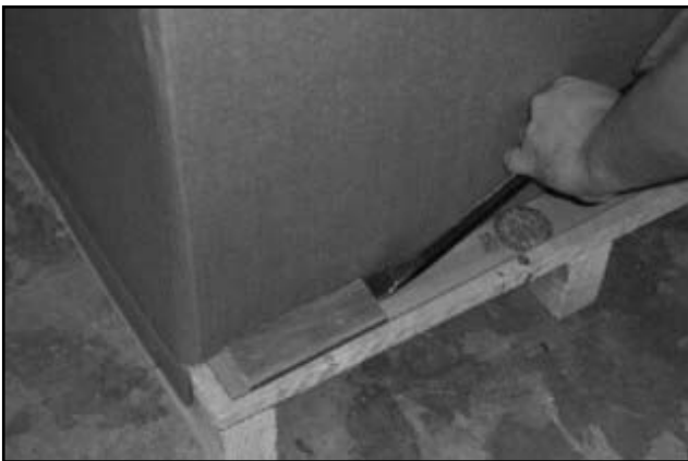
Use a pry bar and mallet to remove the hold-down blocks.
