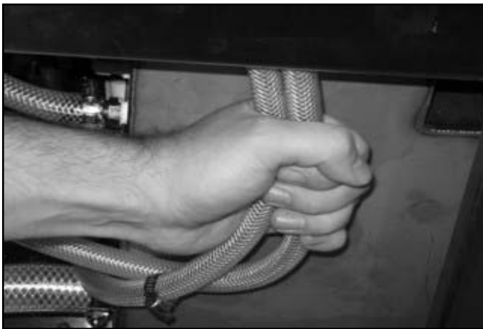
Pulling the discharge hose out.
