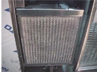
**Step 1:** Locate grease filter on the front of the condenser air in duct.
