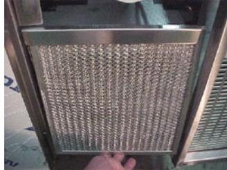
**Step 5:** Pull downwards to release the filter at the top.
