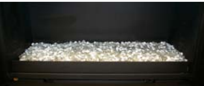
Figure 27c. Completed firestone installation.
