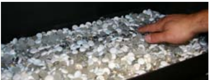
Figure 27b. Spreading the firestones evenly .
