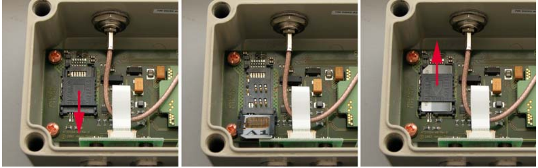
Fig. 4: Installing the SIM card in the A733GSM/GPRS RTU
