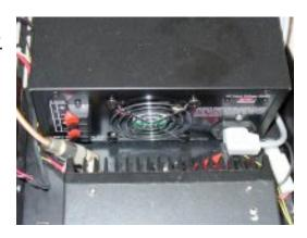
The power supply is positioned so that the front panel attachment lugs do not extend beyond the rack shelf.
