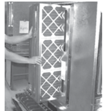
Figure 6: Replace filters – ERV1500i and ERV3000i
