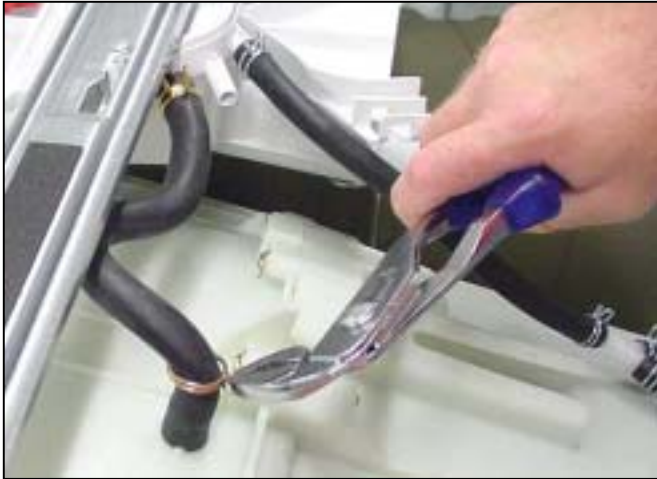
Disconnect dispenser hoses
