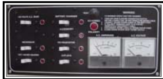
AC Breaker Panel
