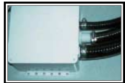
Cabin Drain Sump Pump
