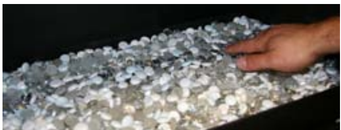
Figure 28b. Spreading the firestones evenly .
