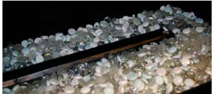
Figure 33. Completed glass bead installation. (Note: place glass beads on top of mesh pilot cover.
