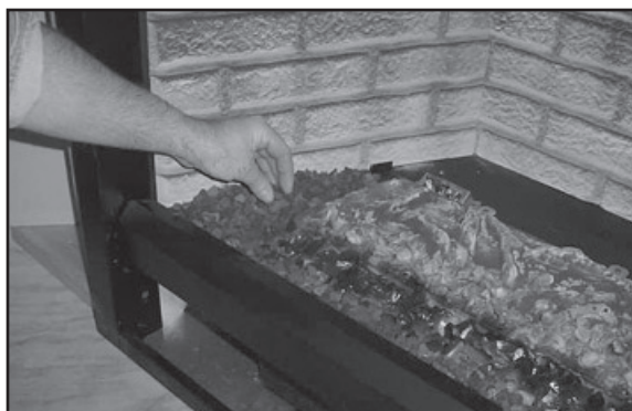
Figure 10.3 Placing the Lava Rock
