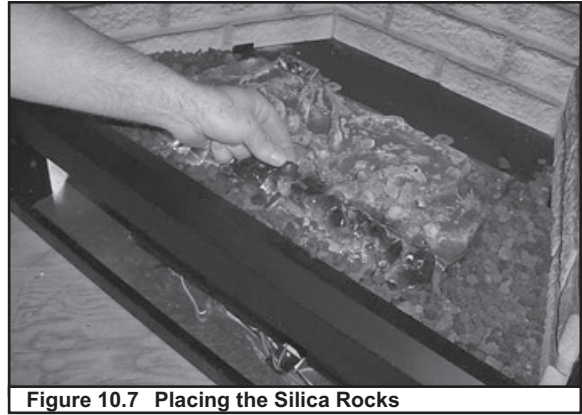
Figure 10.7 Placing the Silica Rocks
