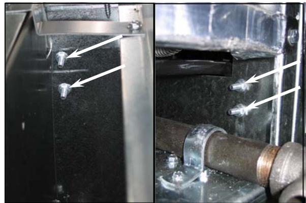
Figure 5. Insert bolts, but do not tighten.
