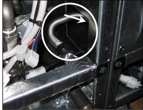
Figure 4. Connect flexlines and align cabinet connection holes.
