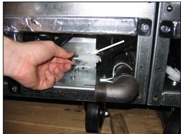
Figure 6. Connect heater-tape harness.
