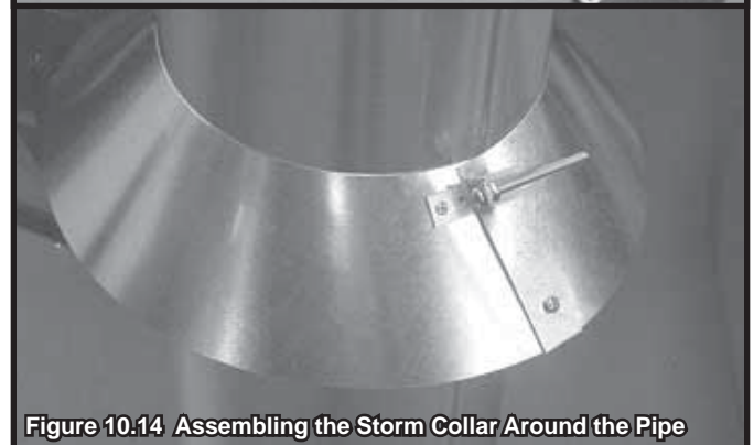
Figure 10.13 Assembling the Storm Collar
