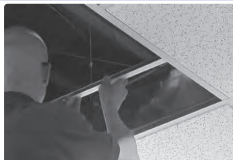
②a Place the T-rails on the T-frame
