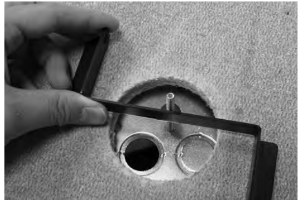
② Attach the Z bracket to the ceiling tile and the back plate.
