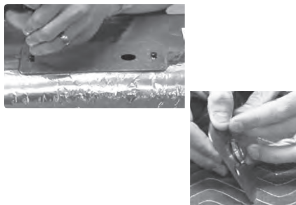
②b Remove terminal cover and attach clamp and ring.
