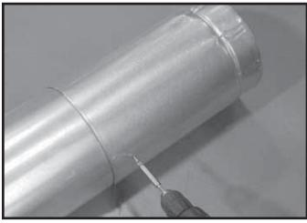
Figure 10.7 Screws into Slip Section
