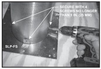
Figure 10.18 Secure Pipe with SLP-FS
