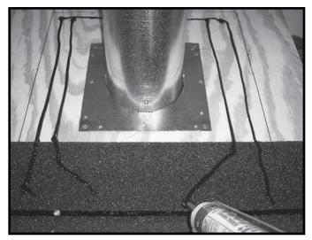
Figure 10.20 Apply Sealant
