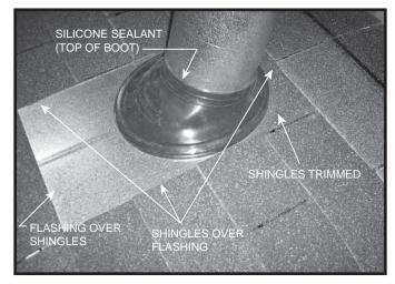
Figure 10.22 Installation Complete
