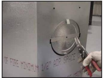
Figure 9.7 Cut the metal retaining band and fold the sides out.
