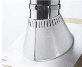
8. Next, slide the storm collar down the chimney until it contacts the flashing. Tighten the nut and bolt and seal the collar to the chimney with a waterproof, non-combustible silicone sealant. Finally, twist on your rain cap and you can head back inside. If the chimney extends more than 5 feet above the roof deck, roof guys with telescoping legs and draw bands are required.
