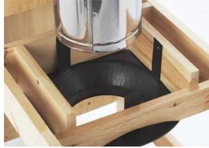
5. Then, from beneath the support, insert the stove pipe adapter and twist-lock it into place.
