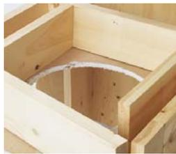
3. To install the ceiling support, just slide the assembly into the framed opening from below. Once you ensure that the finishing plate is flush with the underside of the ceiling and assembly is level, secure it with screws.
