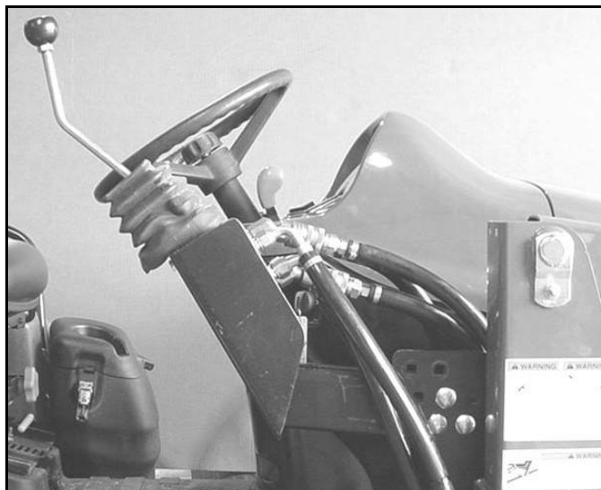
Figure 13. Control Valve Installed
