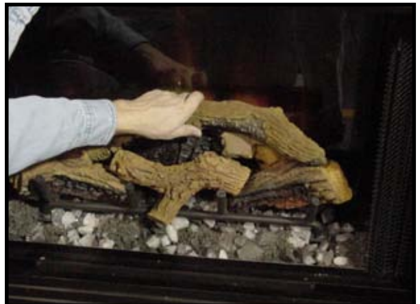
Figure 11 - Replacing Log Assembly
