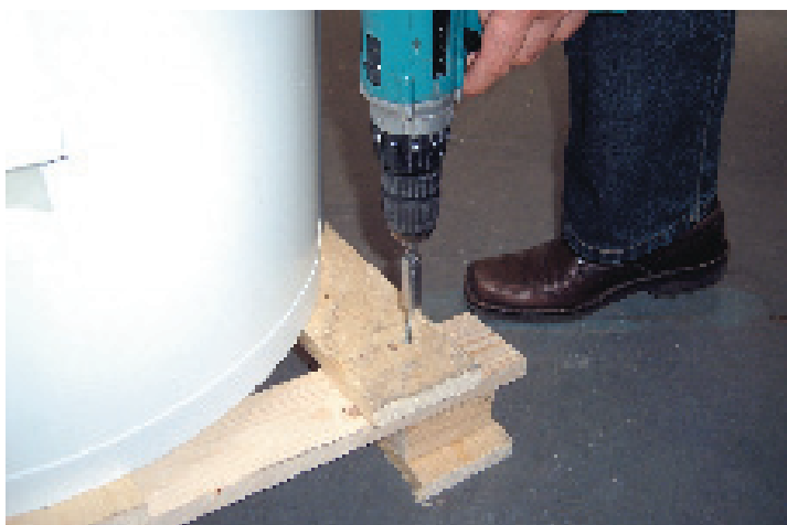
3. Removal of screws
