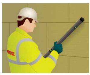
Please note that during stages 8 and 9, the surface of the insulation should be checked for plumb, level and flushness using a long spirit level.
