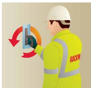
Weather conditions must be closely monitored as the top coat cures through the evaporation of moisture. The temperature must not be below 5°C on a falling thermometer or below 3°C on a rising thermometer (ensuring it rises above 5°C). There must be no risk of frost within 48 hours of application. The finish coat must be suitably protected against rain, strong winds and high exposure to the sun.
