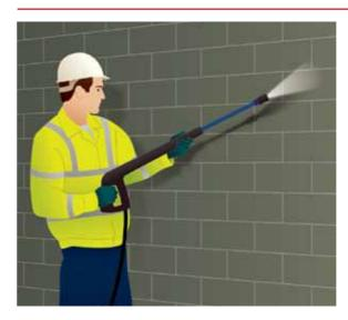
The surface should be thoroughly checked and prepared before any work commences. Walls should be stable, dry and free from dirt, dust, old peeling paint and other contaminants as these will reduce the adhesion of the board adhesive. The ideal method is to wash the entire wall using a pressure washer or mechanically (e.g. using a wire brush). If required, the facade should receive an application of ROCKWOOL Fungicidal Wash.
