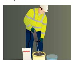
ROCKWOOL Brick Effect Finish should be properly prepared by thoroughly mixing a full bag of the specified finish coat with 4.4 to 5 litres of clean, cool water using a slow rotation drill with a suitable mixer. After achieving a homogenous mix, free from lumps, leave for 5 minutes and then mix again. Once prepared it should be used within 1 hour, mixing every 30 minutes.
