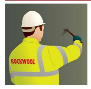
The substrate must be inspected to identify potential problem areas such as (but not limited to) existing loose coatings or uneven surfaces. Where existing render coatings are present these should be checked for loose or blown areas via a hammer test. All identified areas must be removed and made level using a suitable levelling mortar, i.e. ROCKWOOL Anti-Crack Render.
