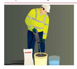
Weather conditions must be closely monitored during the application of the dashing mortar. ROCKWOOL Dash Receiver should be properly prepared by thoroughly mixing a full bag of the specified colour with 4.5 to 5 litres of clean, cool water using a slow rotation drill with a suitable mixer. After achieving a homogenous mix, free from lumps, leave for 5 minutes and then mix again. Once prepared it should be used within 1 hour, mixing every 30 minutes.
