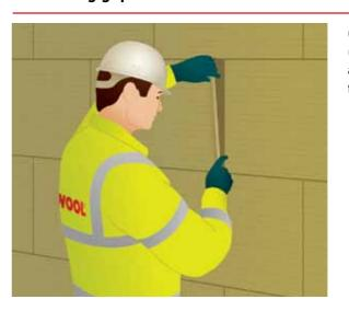
Gaps between insulation boards larger than 2mm should be filled using strips of insulation. Filling of the joints with mortar is not acceptable as this may cause cold bridging and cracking of the finish render.
