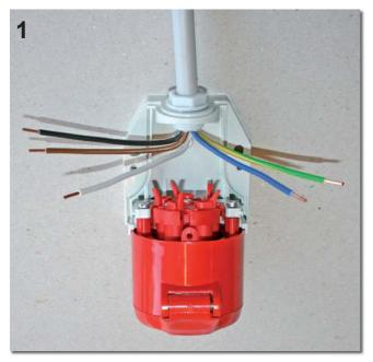
Remove 90 mm of the outer cable sheath and feed it through the grommet into the enclosure. Then strip 8-10 mm of insulation from the wires.
