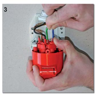
Simply press the release lever to remove wire from its terminal.
