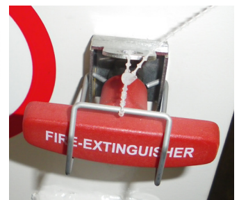
Picture 196. Seal mechanical pull handles
