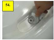
To replace the Trough overflow/seal and nut, loosen the black nut with a 32mm spanner (Pic 55). This will disconnect the tubing from the header tank. Pull up the pipe and replace the overflow fitting (Pic 56)
