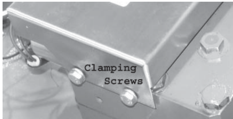
Figure 131. Place Profile or E-Troll Module onto Valve and tighten screws
