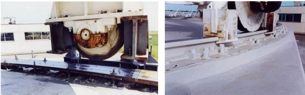
Fig. 2.2 : Installation of the metal plate (antenna lifted) and finished work (the plate and the basement are both white painted)
