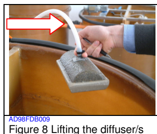
Figure 8 Lifting the diffuser/s
