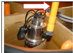
Figure 7 Lifting the motor-driven pump
