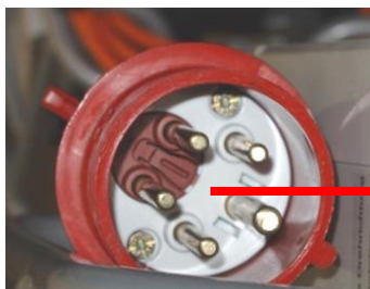
fig1: reverse of the phase (rotation direction pump)
