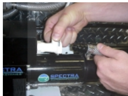
Connecting brine discharge hose
