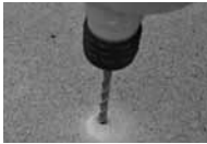
Drill hole using a 8mm / 5/16in drill bit
