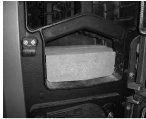
Fig. 4. Position of ceramic catalyst on the exchanger shelves in a KLIMOSZ MULTICOMBI.
