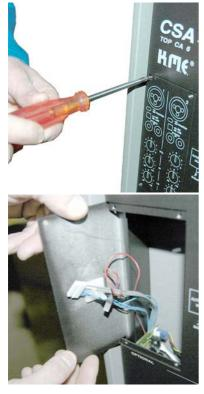
• Remove all cables, especially the power cord, from the CSA 400 D.
