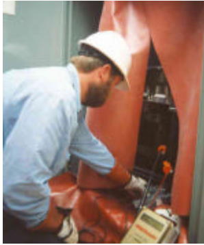
Fig 15 – Use of insulating mats in switchboard application
