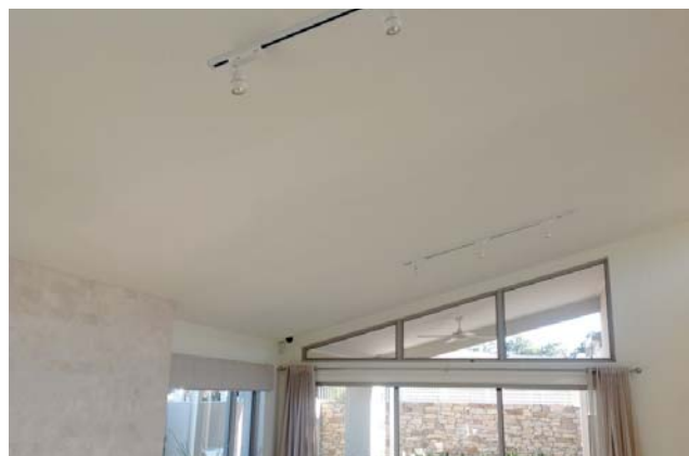
Figure 6: Plasterboard surface under normal lighting conditions
