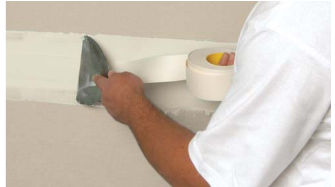
2. First coat - Bed tape
