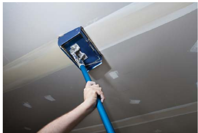
Figure 87: Flat Box Application
