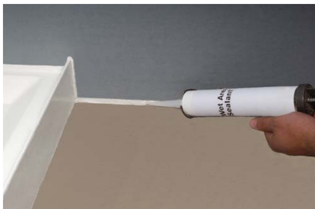
Figure 61: Seal Floor and Wall Junctions
