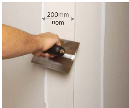
3. Apply second coat to corner faces
