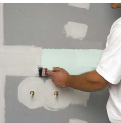
7. Apply two liberal coats of Wet Area SealCote at all joints, junctions, penetrations and fastener heads.
