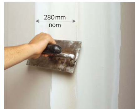
4. Apply third coat to corner faces
