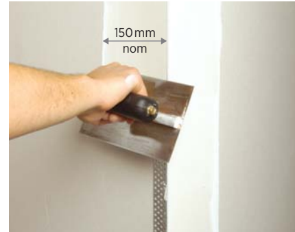
2. Apply first coat to both corner faces
