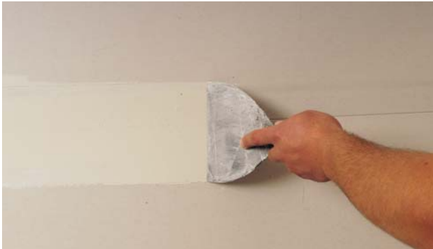
1. First coat - Bedding compound
