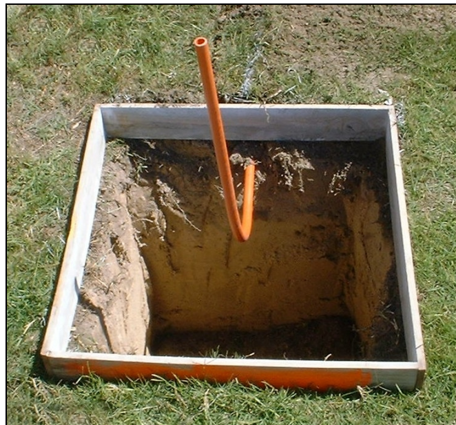
Figure 3-2: Conduit in Post Hole
