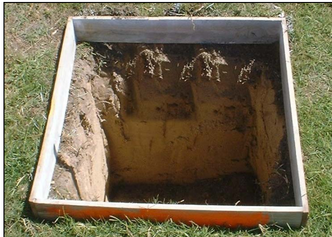
Figure 3-1: Formwork for the Gate Post Footings
