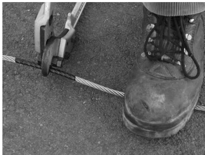
Figure 3-13: Cutting the Main Cable to Length
