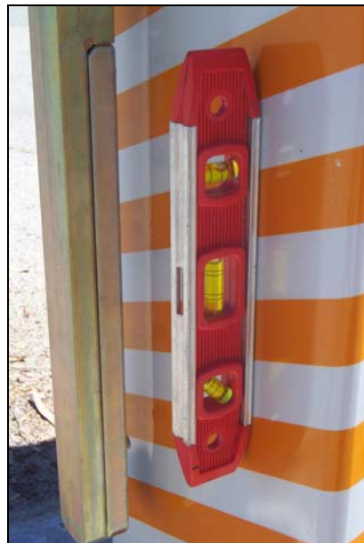
Figure 3-5: Setting the Post Vertical
