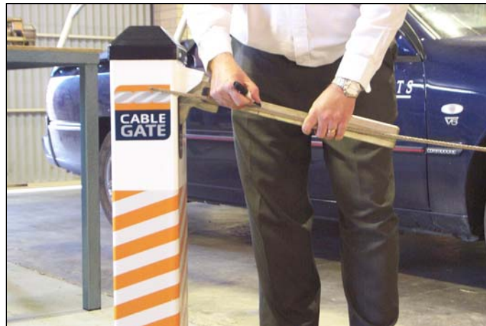
Figure 3-12: Marking the Main Cable to Length for cutting
