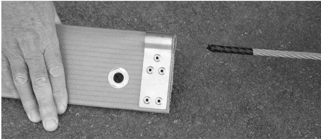
Figure 3-14: Inserting the Main Cable into the Cable Sheathing
