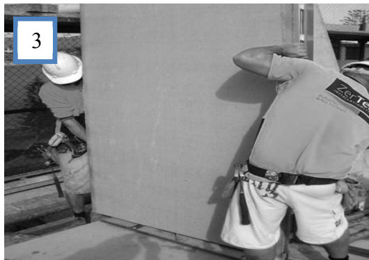
3 Position first panel in line with surveyor's wall starting point. Note: For XL Thermal Panel - ensure insulation is to correct facing side of the panel
