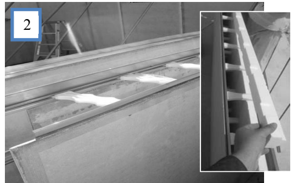
2 For increased speed of panel installation fix the panel joiners to the panel before erecting. NOTE: For XL Thermal Panel – fix the insulation infill and secure using the galv nails
