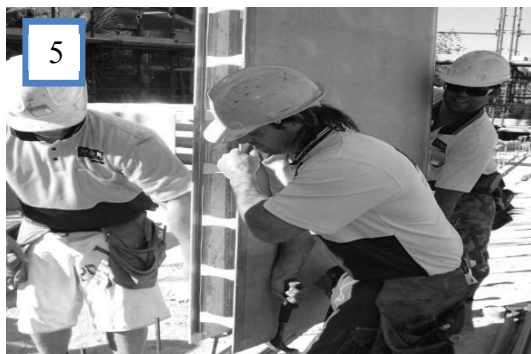
5 Standard panel requires three people to be placed into position.
