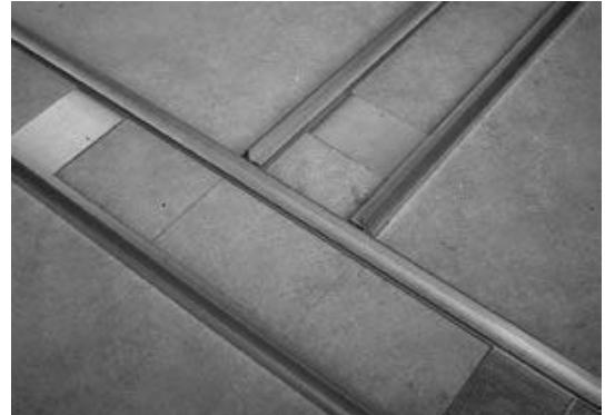
Fix bottom plate assembly to set out on slab with 20mm masonry pins.
