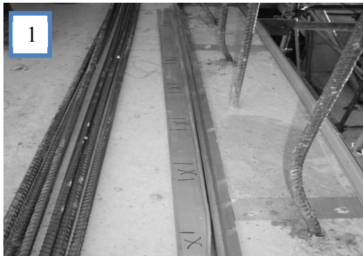
1 Create jig to ensure starter bars do not conflict with studs
