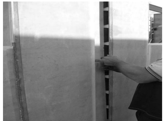
Place Tee Closure into position ready for closing off
