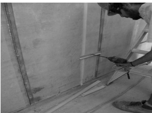
Fix a toggle (ply wood or aluminium angle) to the tee junction bringing it flush with adjacent panels.
