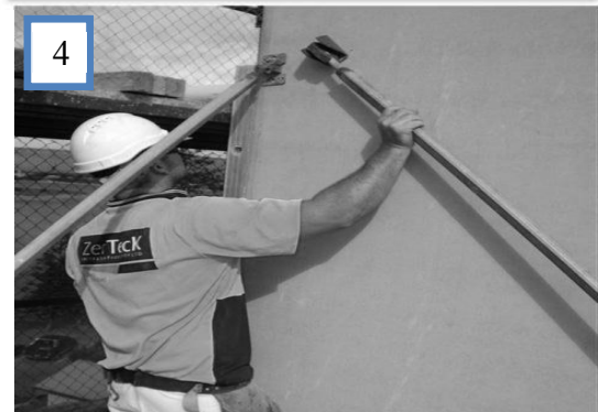
4 Secure brace foot plate to slab with Excalibur bolt and brace to panel with self-tapping screws into panel stud. Proceed to plumb panel in all directions utilising the brace's push pull mechanisms and a level.
