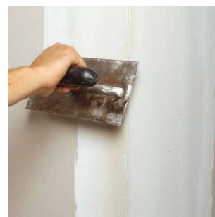
Step 4 – Apply 280mm third coat to corner faces
