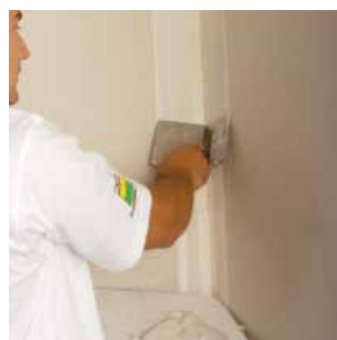
Step 4/5 – Apply second coat & sand
