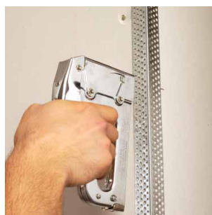
Step 1 – Cut angle and fix to both sides of corner @ 300mm
