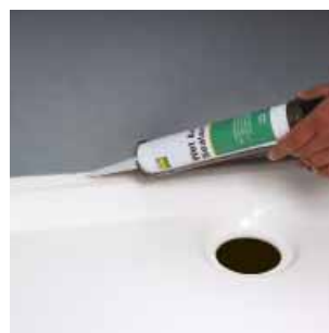
Figure 63 Seal sheet edges over baths, shower bases, laundry tubs
