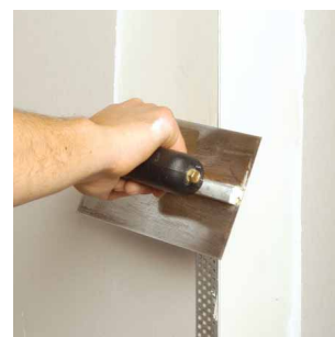
Step 2 – Apply 150mm wide first coat to corner faces
