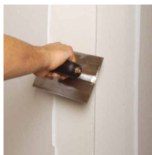
Step 3 – Apply 200mm wide second coat to corner faces
