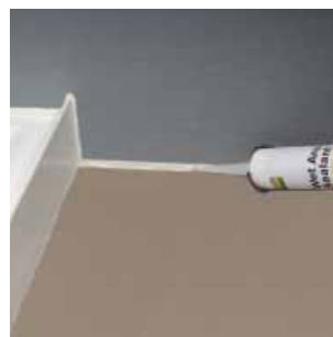
Figure 64 Seal floor and wall junctions
