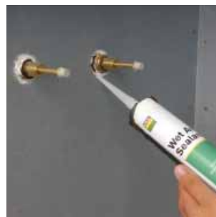
Figure 62 Seal penetrations
