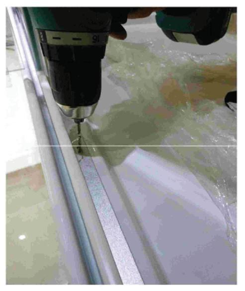
Then screw the bottom bar just like the corner strips with screws + caps. if necessary, can be sealed with silicone under the bottom bar..
