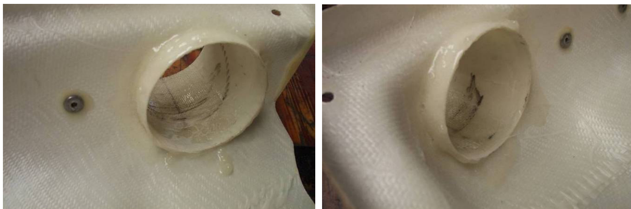
Figure 34. Air Filter Box Plumbing – Incorrect
