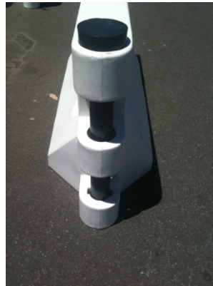
LINK PIN IN POSITION
